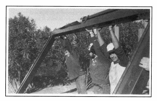
If the fork lift is available, power posts may be set upright and POWER BEAM lifted and set in place.
