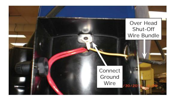
Now you are ready to connect the Push Button "UP" wire to one of the 2 wires remaining in the overhead shut off wire bundle. Remove Push Button "UP" wire from terminal **3L2**. Cut some length off of the wire. Wire nut the Push Button "UP" wire to one of the 2 remaining over head shut off wires.
